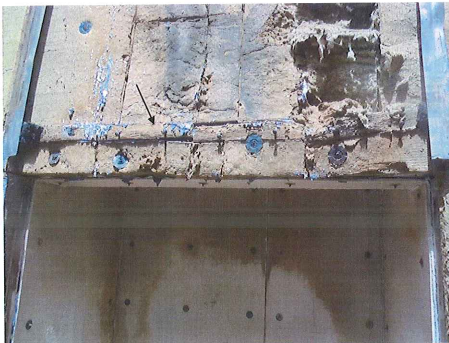
Cavity barrier at the top of combustion chamber
