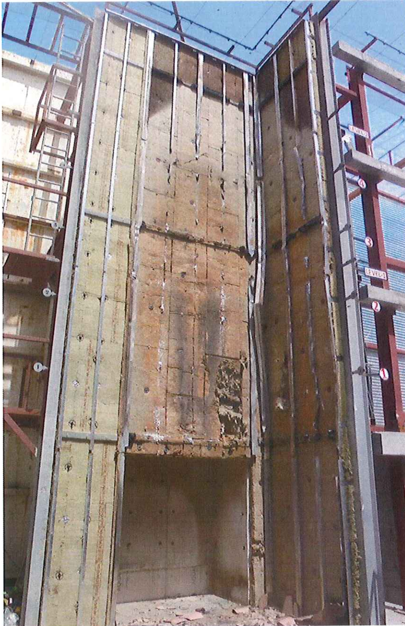
Cavity barriers, insulation and railings
