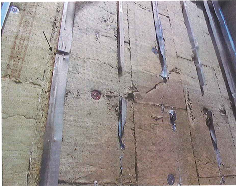
Vertical cavity barrier, insulation and railings
