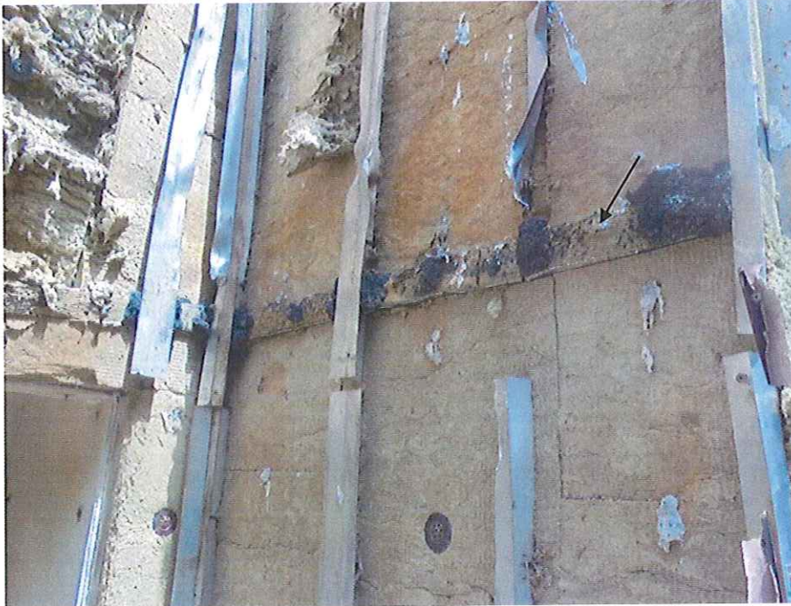
Cavity barrier on wing wall
